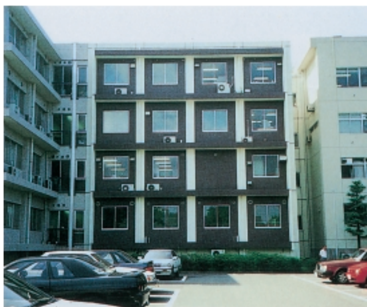
The 3rd and 4th extension building including Information and Reference Center of Tropical Medicine, The Institute of Tropical Medicine, Nagasaki University
